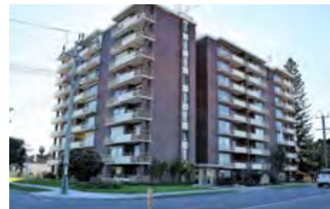
Higher density apartment building, Wembley
