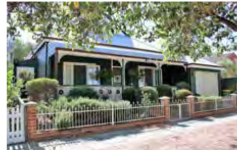
Medium density pre-war cottage detached dwelling, West Leederville
